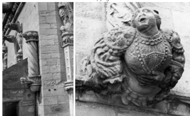
Figure 37: Detail of the south-east angle of Stirling Palace in 1900 (left), and decorated shaft corbel (right). Crown Copyright: Historic Environment Scotland
